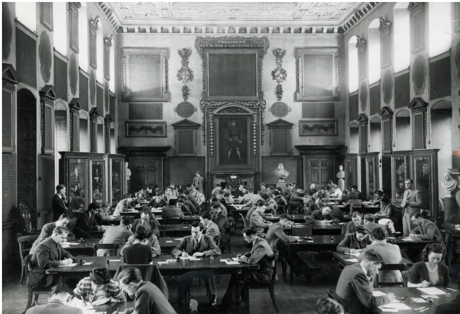
Examinations in the Great Hall, St Bartholomew's Hospital, 1960s
